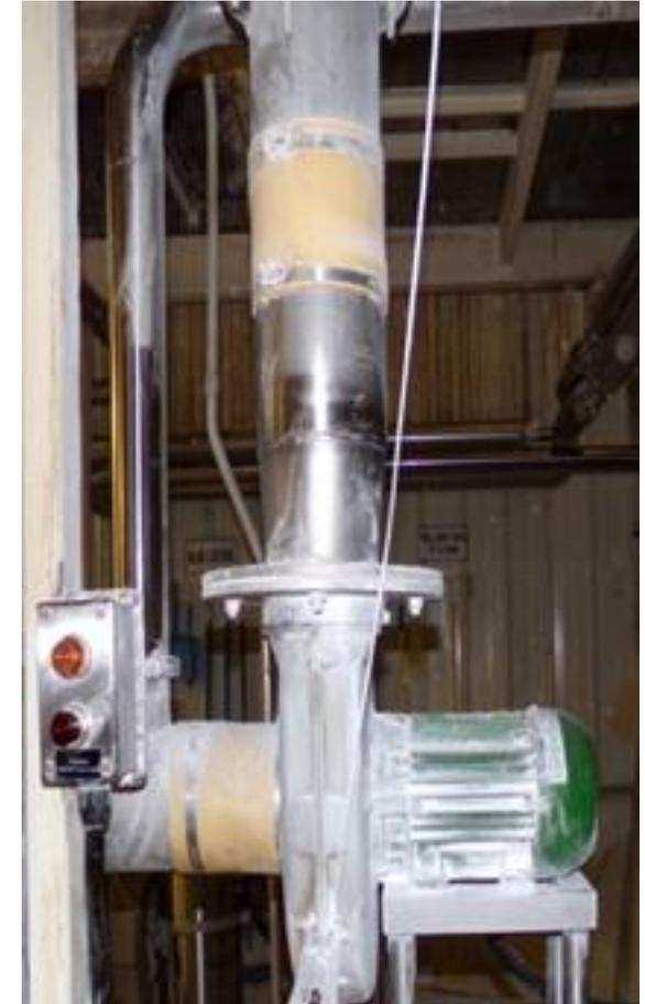
BFM connections with complete **seal** vs. **clamped** connections that develop niche or powder ingress / egress. These can also be used for CIP return connections and sampling.
